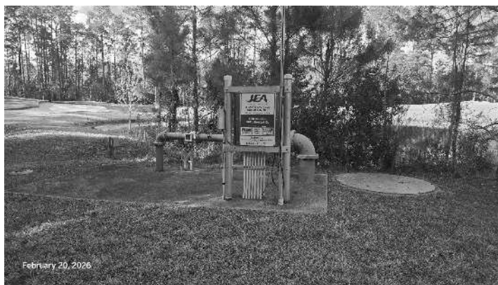
Field Photograph of JEA Re-Use Delivery Point
